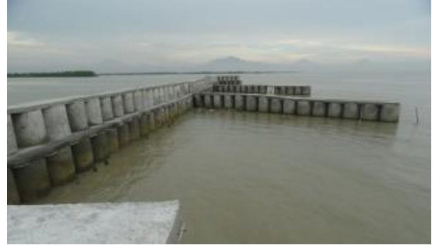
Figure 5: Breakwater of concrete buis type built on 2012.
