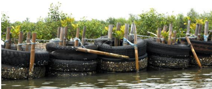
Figure 3: Breakwater of tires bambo combination type in study area.
