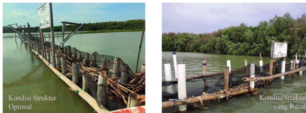
Figure 6. Permeable breakwater structural damage condition
