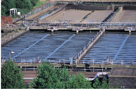
Figure 3.5 Industrial scale of horizontal gravity filter
