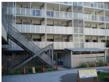
Fig. 5 Kobe municipal housing in HAT Kobe area, Kobe, Japan. Source : field survey, 2012
