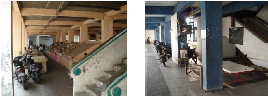
Fig. 13 The absence of elevators makes the elderly who live in the upper floor have to find the common facilities in the ground floor by stairs. Source : field survey, 2012
