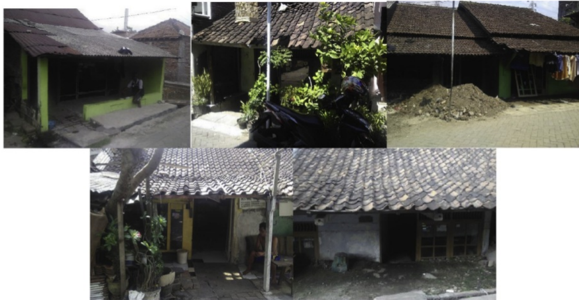
Fig. 5. Sinking houses affected by the increased street level.
