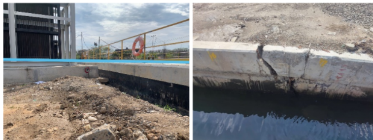
Figure 7. Structural damage and structural settlement
