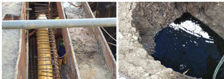
Figure 9. Existing pipe leakage
