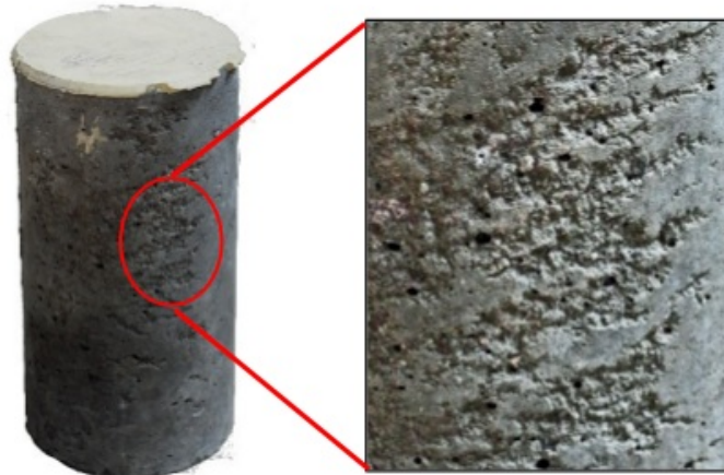
Fig. 4. Poor compacting due to low workability for 10M specimens.
