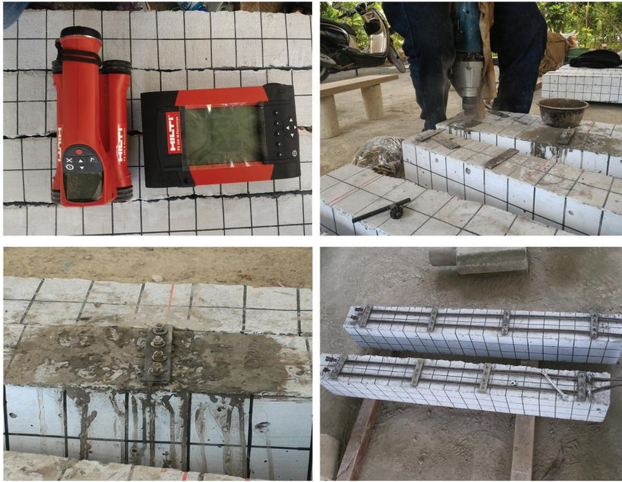
**Figure 3.** Strengthening process involved the location of the current reinforcement to be determined through rebar scanner, drilling, dynabolt and steel plate installed as the end-anchor, steel wire rope installed and dynabolt tightened (Haryanto et al. 2018).
