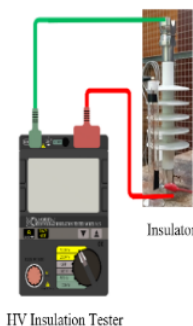
Figure 2. The measuring of insulator resistance
