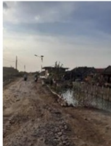
Figure 2. Back road filling
