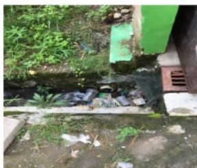
Figure 2. The drainage channel clogged with garbage.
