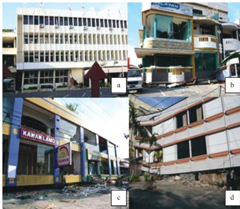
FIGURE 2. The Padang earthquake on September 30 & October 1, 2007: a). The Office of DPU Padang experienced a soft story on the 1 st floor but it was still survived, b). The shophouse 3 stories experienced severe a soft story at the 1 st floor. This floor collapsed, and the 2 nd & 3 th floors fell on it, c). & d). The commercial building experiencing a severe soft story at the 1 st floor. This floor collapsed, and the 2 nd & 3 th floors fell on it (source: http://www.perencanaanstruktur.com/2010/10/bentuk-keruntuhan-bangunan-saat-gempa.html ).
