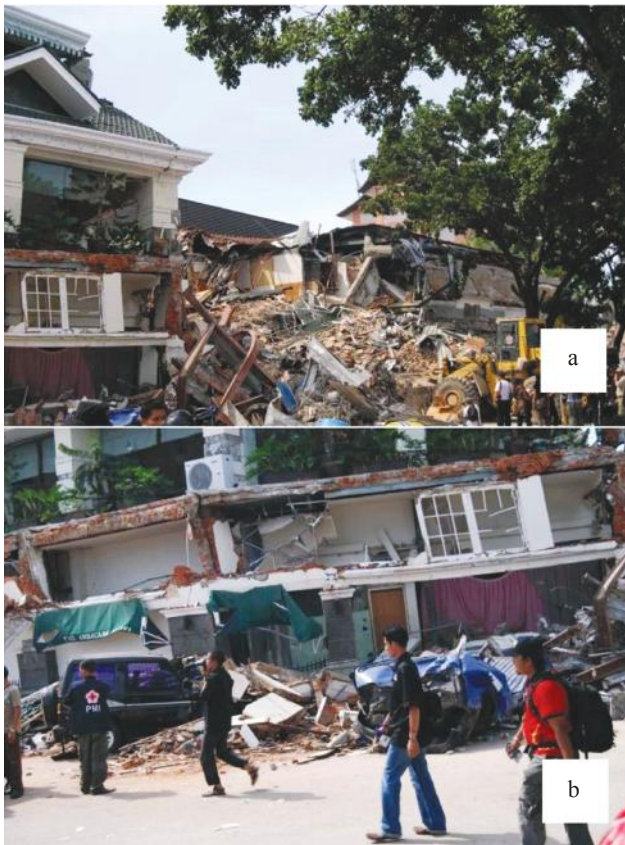
FIGURE 5. West Sumatra Earthquake in 2009, Hotel Ambacang suffered 'sandwich' collapse (source: http://xa.yimg.com/kq/groups/17587015/808630997/name/Kerusakan+Gedung+-+GB+Padang.pdf ).
