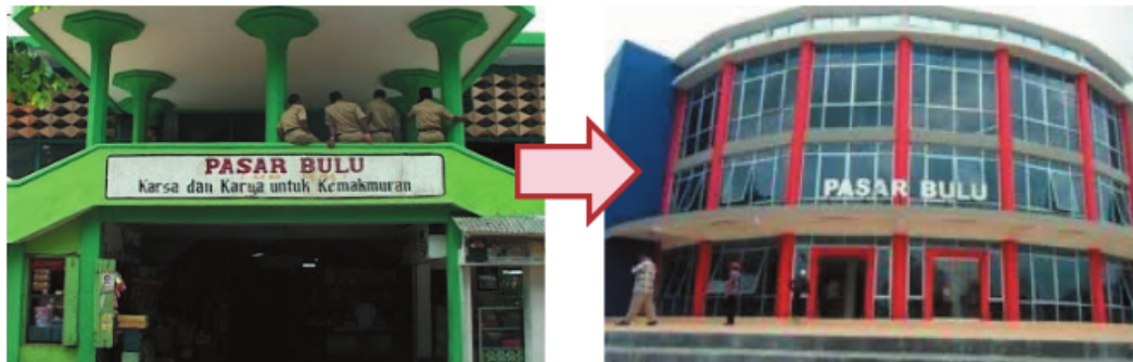
Figure 3. Bulu Market pre-revitalization (left) and post-revitalization (right).
