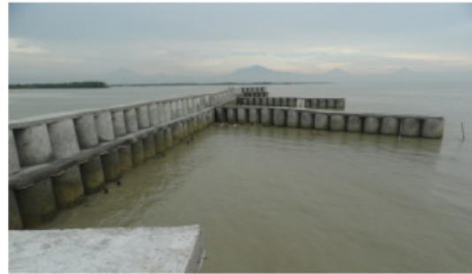
Figure 5: Breakwater of concrete buis type built on 2012.
