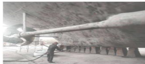
Gambar 5. Proses Sandblasting KMP. Doro Londa
