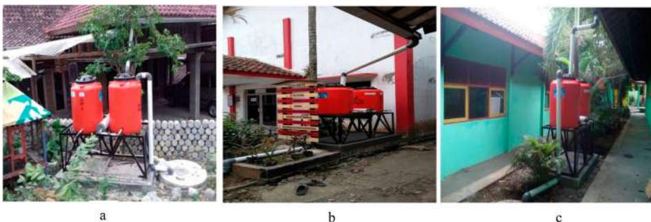
Figure 1. RWH pilot project in public facilities. RWH at Local Government Office – Rowosari subdistrict (a and b) and at State Junior High School 42 Semarang (c). Source: dlh.semarangkota.go.id.
